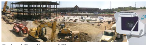
Federal Courthouse, MS
