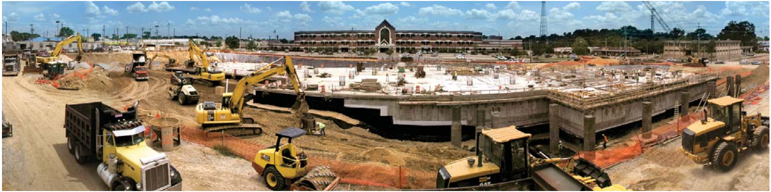
Federal Courthouse, MS
