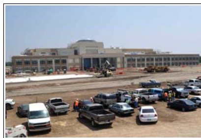
Hays County Government Center, TX
