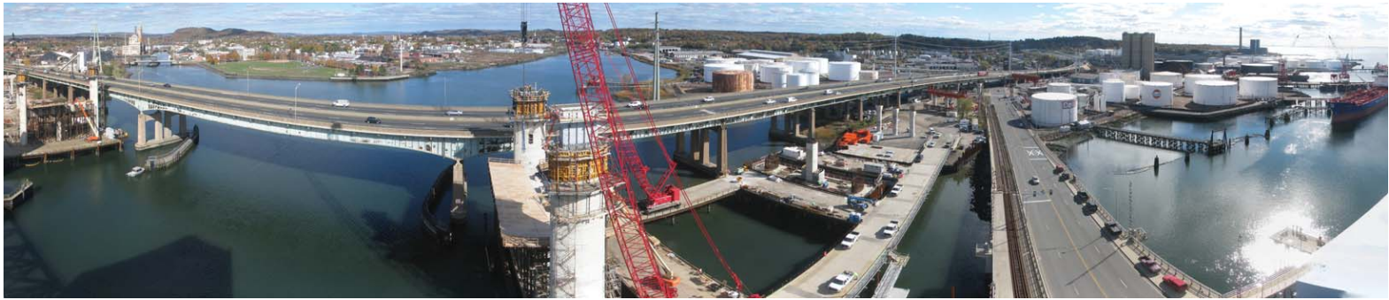
Pearl Harbor Memorial (Q) Bridge, New Haven, CT
